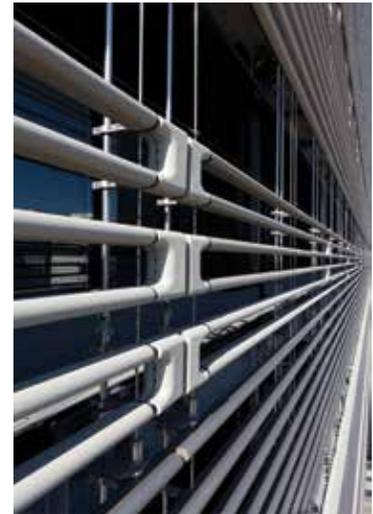
Figure 14. A close-up view of the ceramic transpiration system built into the NBF Osaki façade, known as BioSkin. © Harunori Noda
