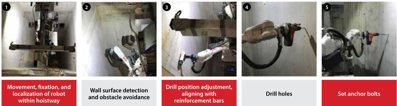
Figure 9. The operating process of R.I.S.E. (Robotic Installation System for Elevators). © Schindler
