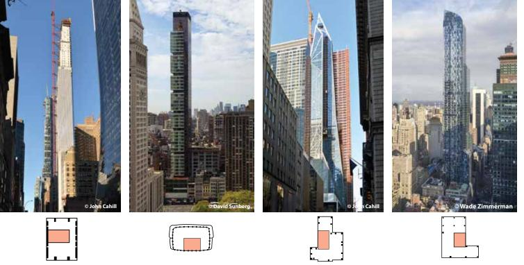
Figure 6. The increasing trend toward superslim towers in New York has affected core position and plan form. From left to right: 111 West 57th Street, 2019; One Madison Park, 2010; 53 West 53rd, 2019; and One57, 2014.
