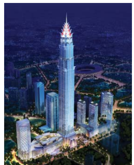
Figure 8. Jakarta is set to contain the world's 5 th tallest building, the 638-meter Signature Tower Jakarta © SRSS
