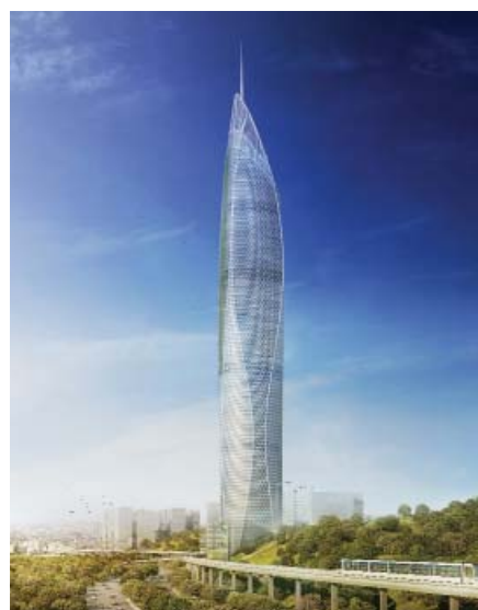
Figure 7. Seoul Light DMC Tower will become a landmark for the city's skyline © SOM / Giroud Pichot
