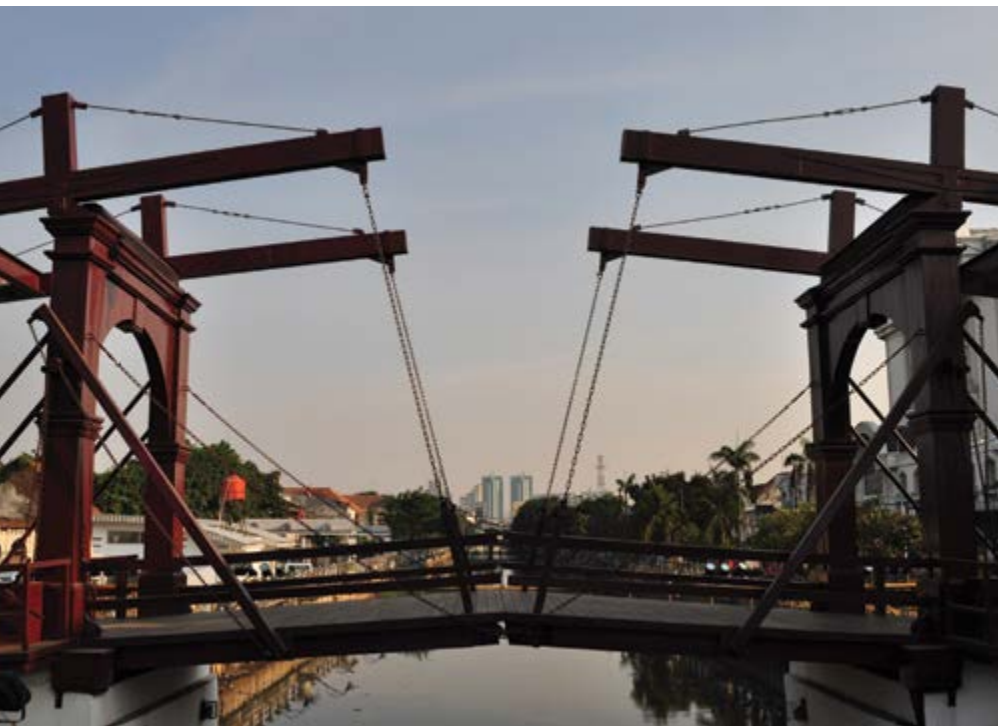
Figure 9. Kota Intan bridge along Ciliwung in Kota Tua (old town). © Thierry Falise
