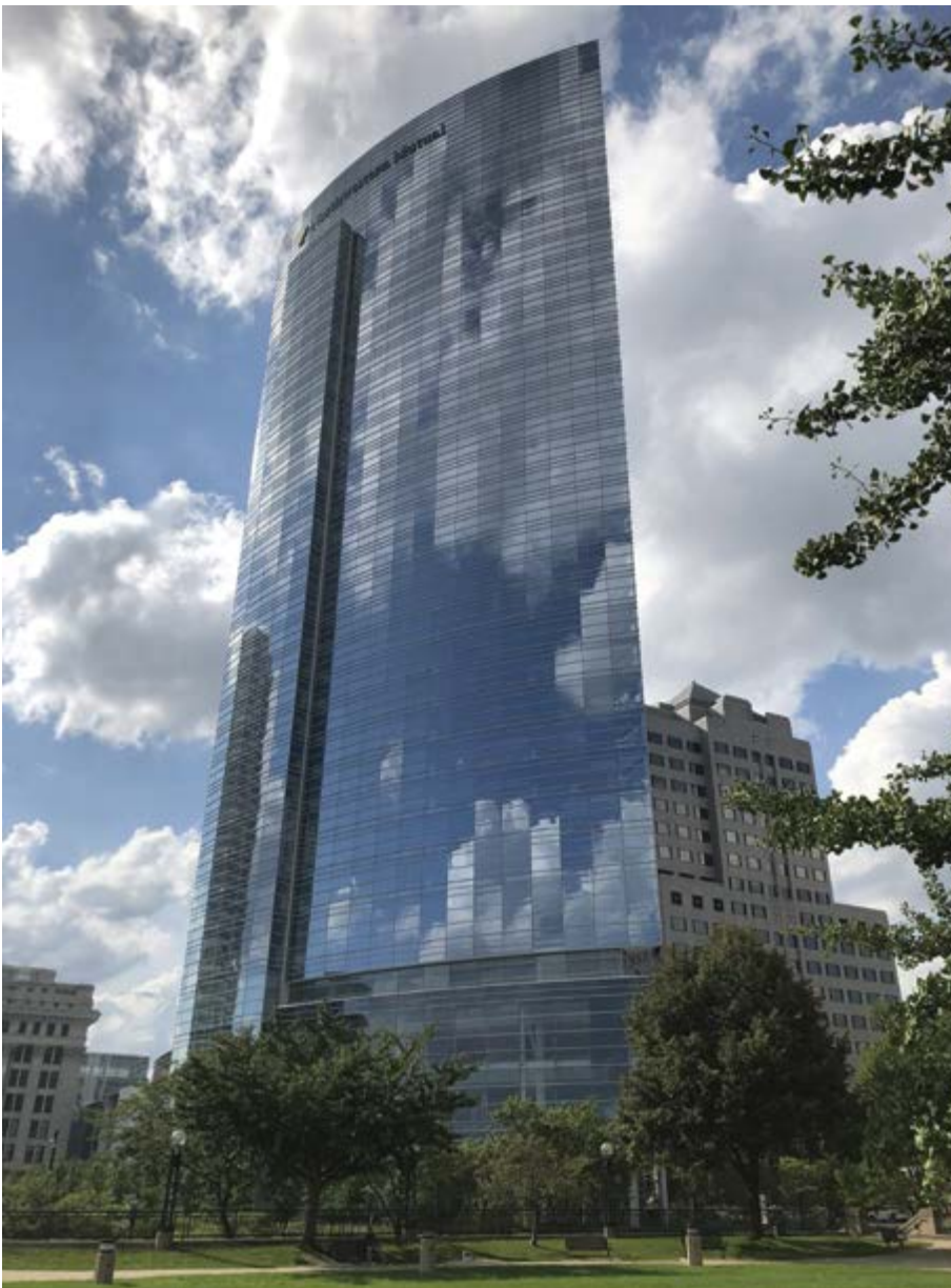
Figure 8. Northwestern Mutual Tower and Commons, Milwaukee, employed high-strength ASTM A913 Grade 65 (450) steel to reduce the amount of material required to meet the loading demand on the steel gravity frame. © ArcelorMittal (Rob Caroti)
