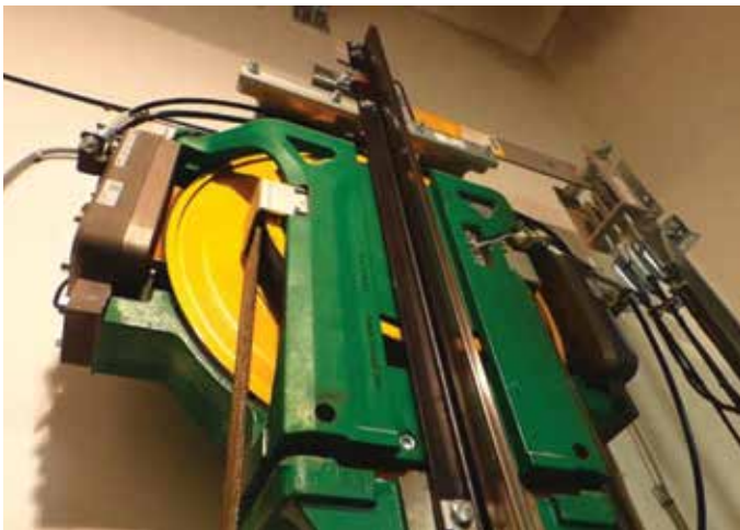
Figure 7. Permanent Magnet Synchronous Motor (PMSM) technology used by an MRL elevator. © KONE
