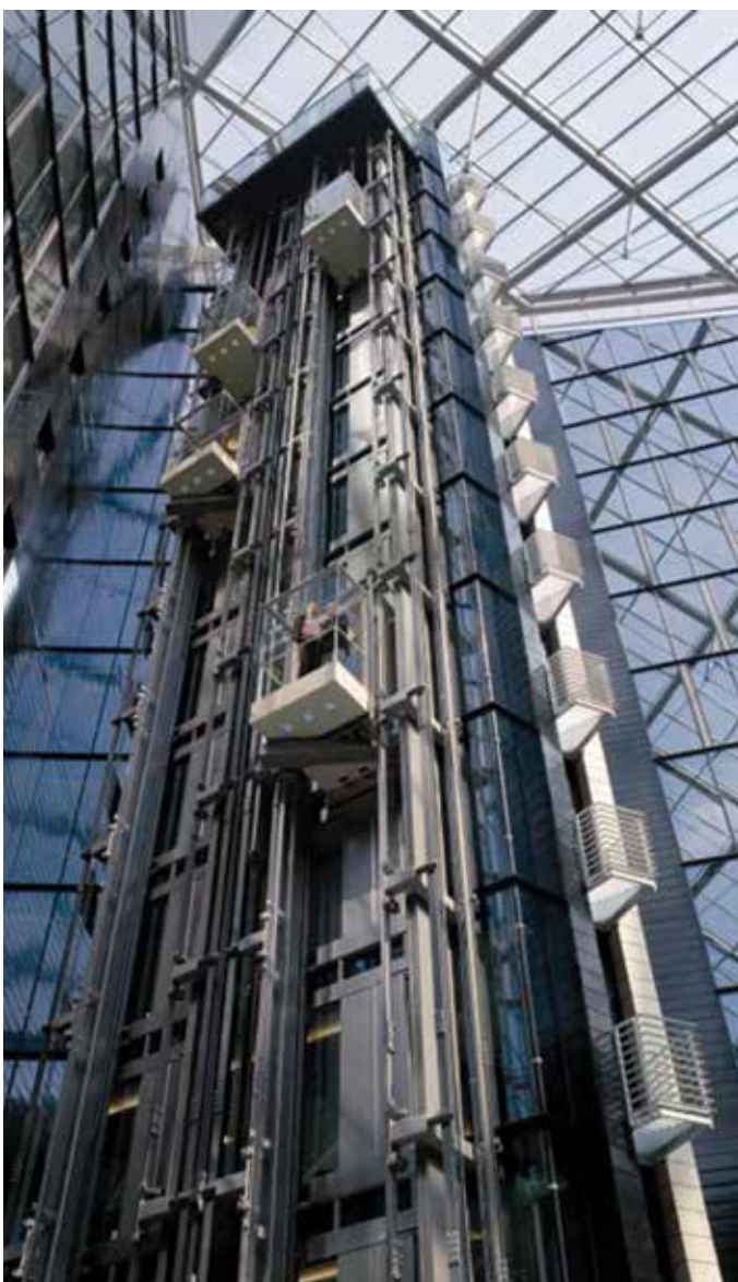
Figure 8. The TWIN elevator system could accommodate two elevator cars in a single shaft, reducing the amount of space dedicated to elevator shafts in a tall building. © thyssenkrupp
