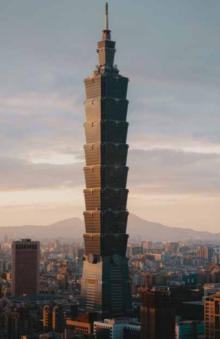
Figure 5. TAIPEI 101—the main body of the tower consists of a stacking of discretely individual, self-contained blocks. © Jon Fobrant
