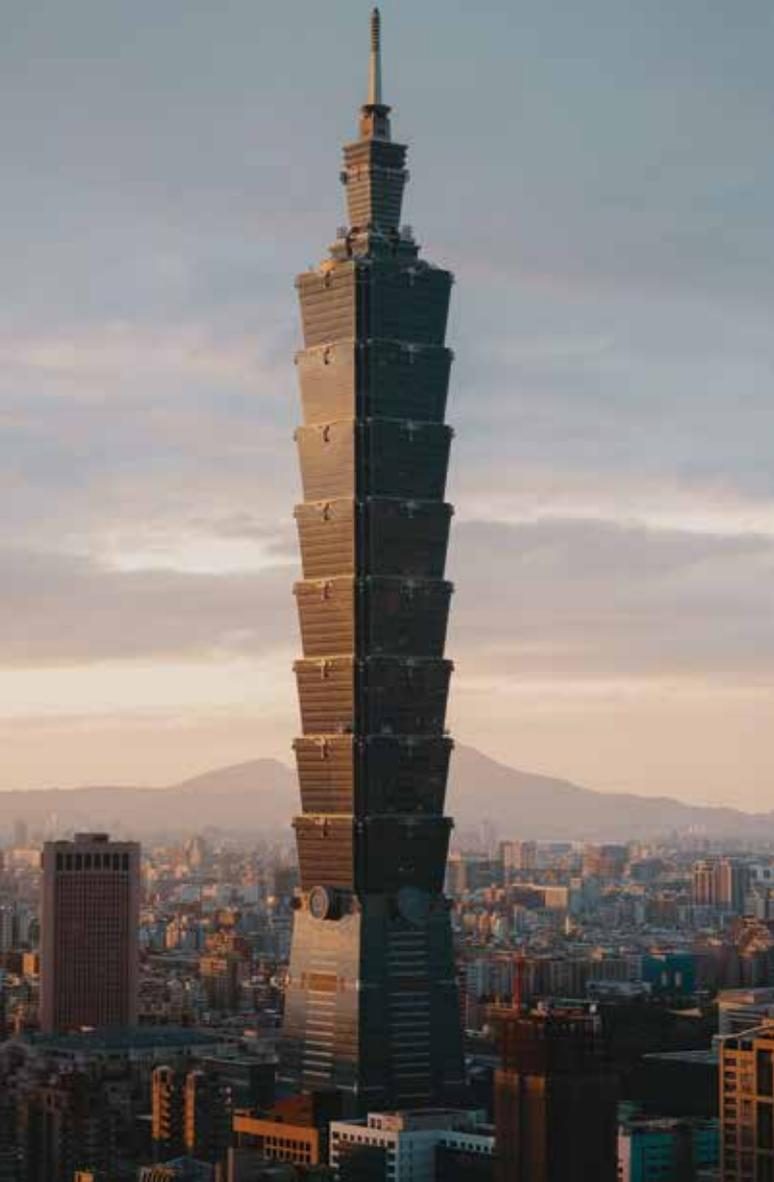
Figure 5. TAIPEI 101—the main body of the tower consists of a stacking of discretely individual, self-contained blocks. © Jon Fobrant
