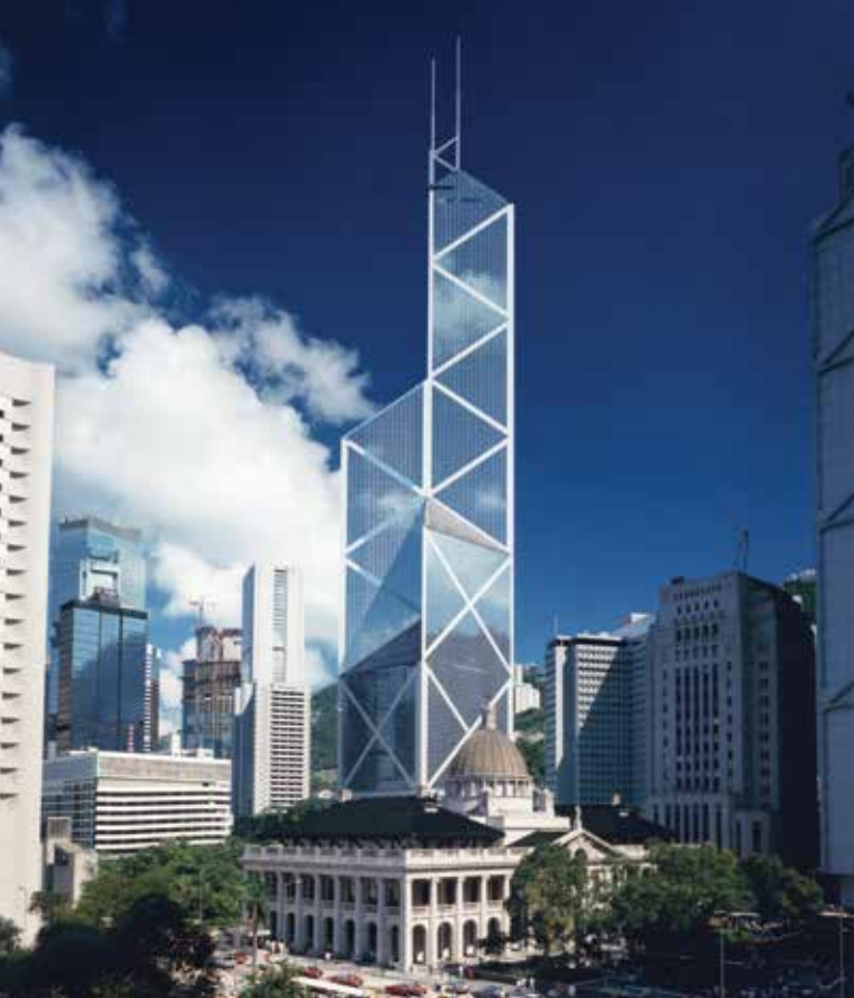
Figure 1. Bank of China Tower, Hong Kong—all of its lateral load-resisting system are on the perimeter. © Terri Meyer Boake
