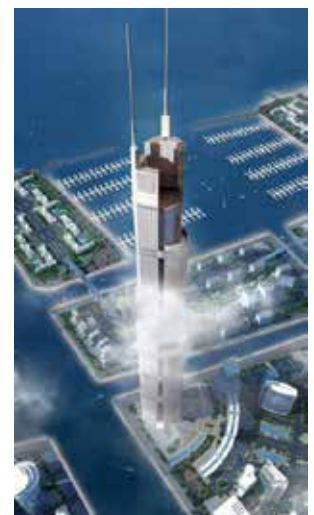
Figure 8. Al Burj, Dubai, there are trusses in the vertical slots “zipping” the legs together, thereby making the three sections of the tower act as one. © Pei Partnership Architects
