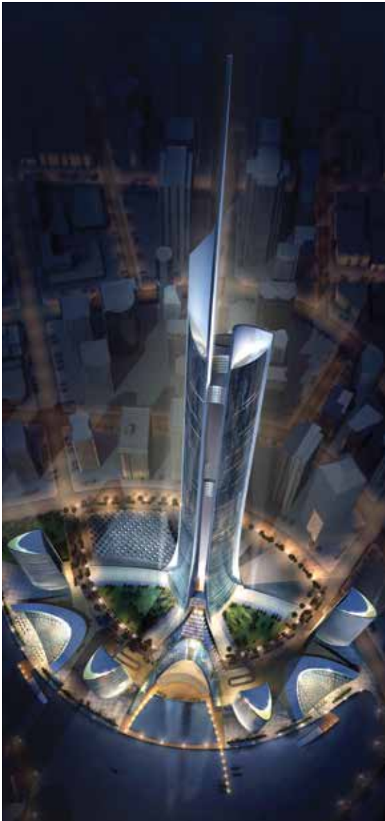
Figure 10. Kingdom Tower competition design, Riyadh—a gently tapering profile efficiently reduces wind loads on the building. © Kohn Pedersen Fox Associates
