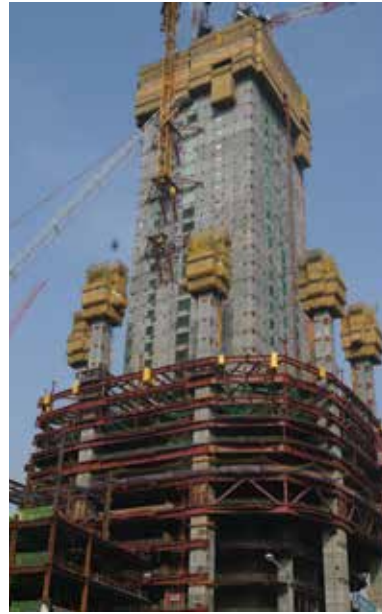
Figure 6. The primary lateral load-resisting system for Lotte is the concrete shear walls at the services core. © Lotte Group
