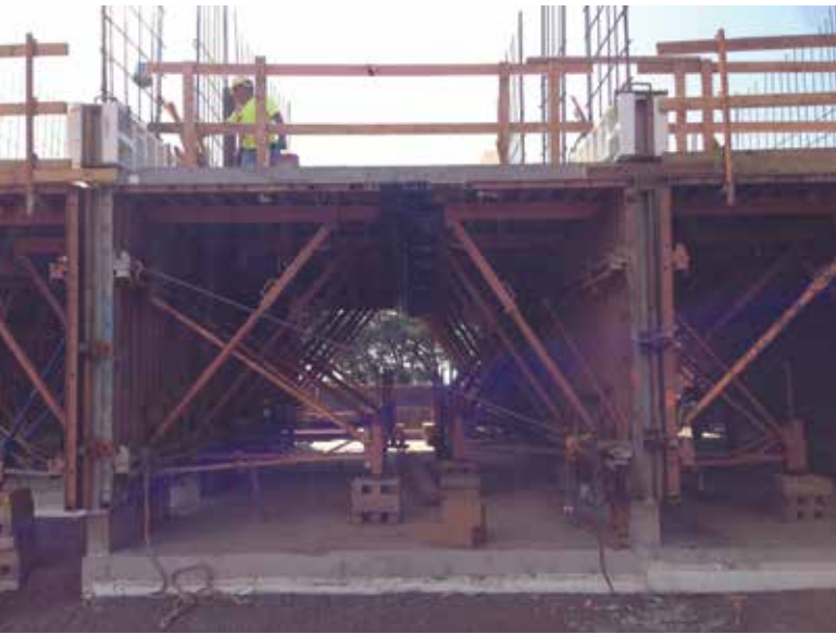
Figure 4. Close-up of tunnel form. © Steven Baldrige
