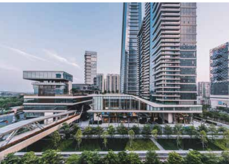
Figure 7. Rather than stacking the towers upon a podium, the design pushes all the retail functions to the perimeter, and brings the towers down to the ground.
