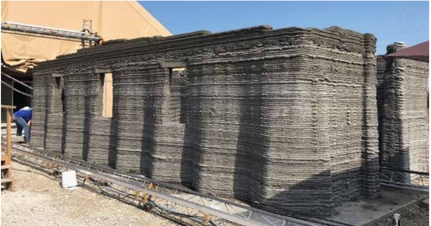
Figure 3. A 3D Printing is seen as a “robotic” application to architecture, but a 3D printer is just a machine, as it has no “intelligence.” Also, it is probably not promising as a technology: commercial buildings are more complex than a pour of concrete (the picture shows a military barrack).
