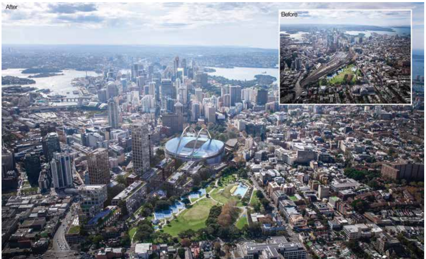
Figure 8. Sydney Stadium, before and after—embedding a stadium in the fabric of the city creates an urban spectacle, enhancing the experience of attending events. © Bates Smart Pty Ltd.
