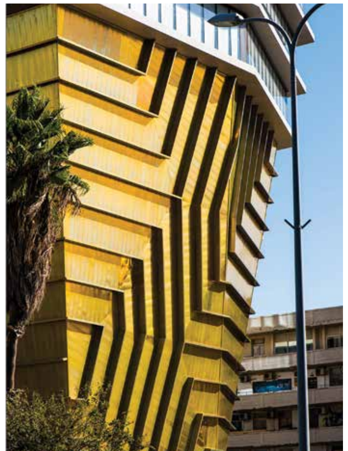
Figure 12. South "leg" cladding. © Ron Arad Architects, courtesy of Asa Bruno
