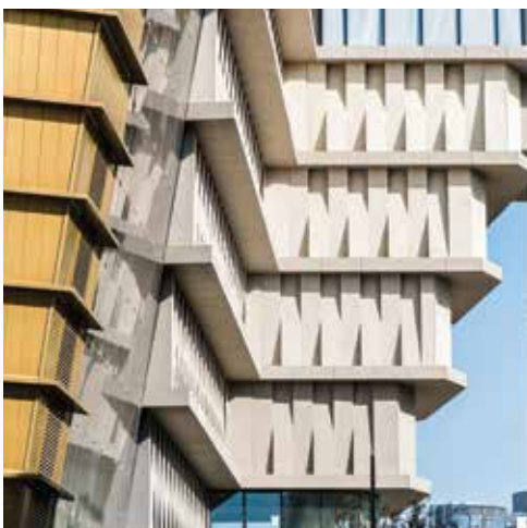
Figure 6. The ventilating “X”-panel. © Asa Bruno
