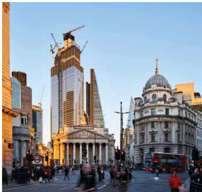
Figure 1. View of 22 Bishopsgate from Bank Junction in London. © Michel Denancé
