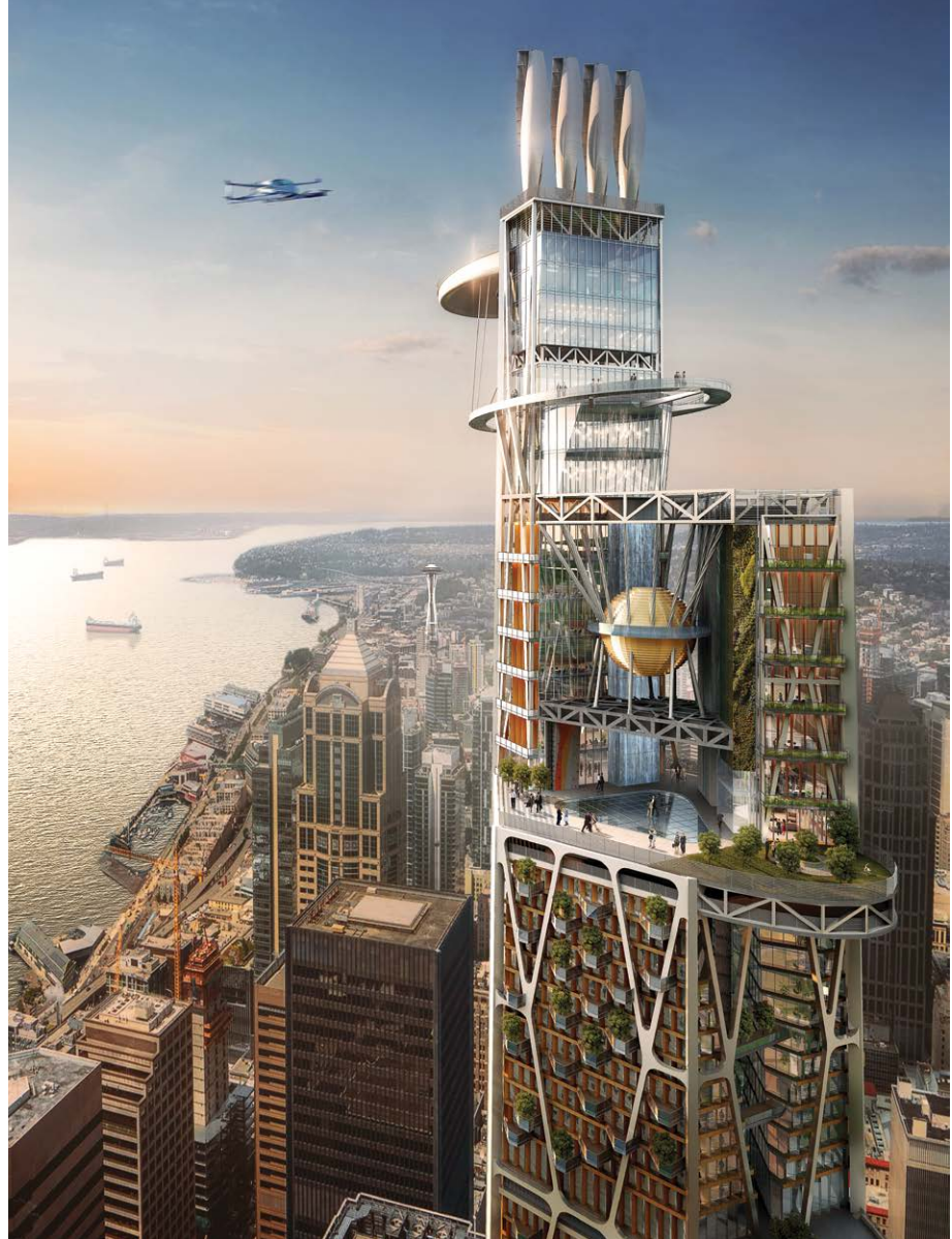
Figure 5. The tower’s pinnacle includes a glass-floored observation deck, a tuned mass damper on display, a perimeter “cloud walk”, and a skyport for vertical take-off and landing vehicles. © 3MIX
