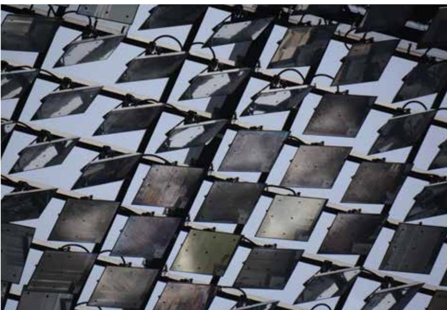
Figure 3. The heliostats on One Central Park, Sydney, provide hours of sunlight and heating to areas normally shaded.
