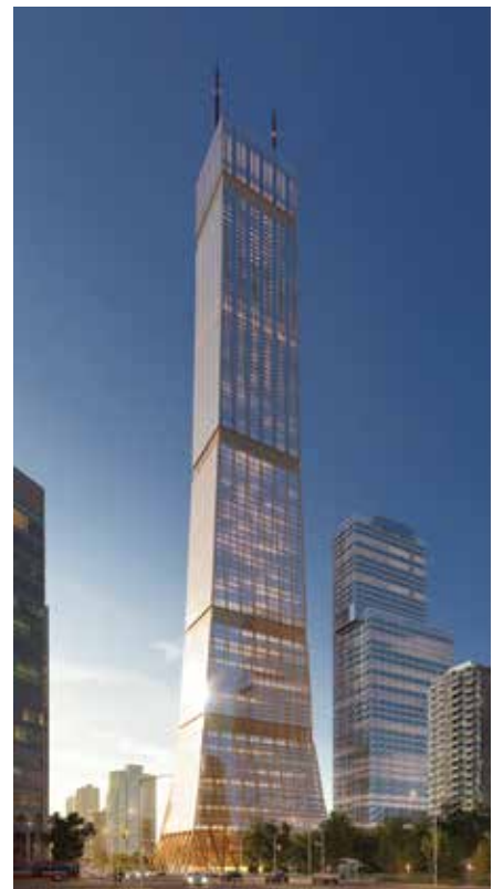
Figure 1. Street view of Hybrid Timber Tower, Toronto, looking north at dusk. This supertall zero-carbon hybrid timber building prototype is designed with a concrete core and diagrid steel external structure, and leverages energy efficiency, smart technologies, façade-integrated photovoltaics (PV), and a district energy cogen plant, combined with an algae bioreactor, to achieve zero operational carbon on-site.
