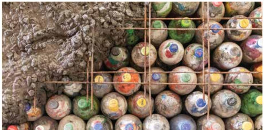
Figure 5. In this configuration, ecobricks purely fill a void, as the surrounding concrete provides overall support. A reference-193 (1.93 kg/m<sup>2</sup>) steel mesh was placed on top of the ecobricks to hold them in position, preventing them from moving when concrete was poured, and to control and limit surface cracking.
