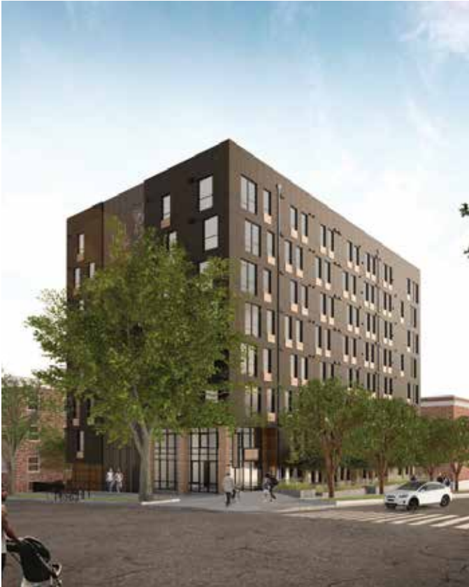
Figure 2. Heartwood, an eight-story mass timber affordable housing project, is underway in Seattle. © atelierjones
