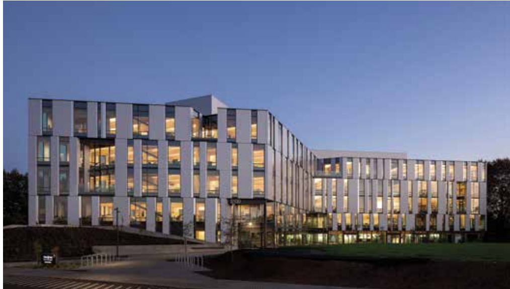
Figure 1. First Tech Federal Credit Union, Hillsboro, Oregon (2018), was the first mass timber project constructed by Swinerton Mass Timber, which would become Timberlab. © Jeremy Bittermann
