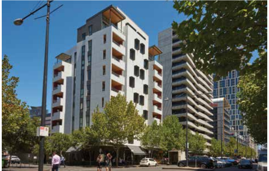
Figure 1. Forte', a 10-story, 32-meter concrete-timber hybrid building completed in Melbourne in 2012, cut its emissions by more than 66 percent by strategically using timber instead of concrete in its structure. © Lendlease
