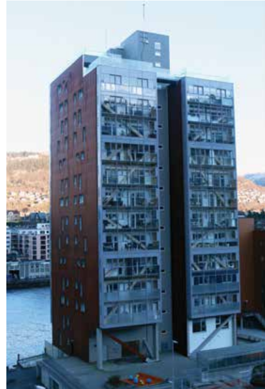
Figure 7. Treet, Bergen, Norway, is the second-tallest all-timber building in the world currently, standing at 49 meters and 14 floors. © Sparrow (cc by-sa)
