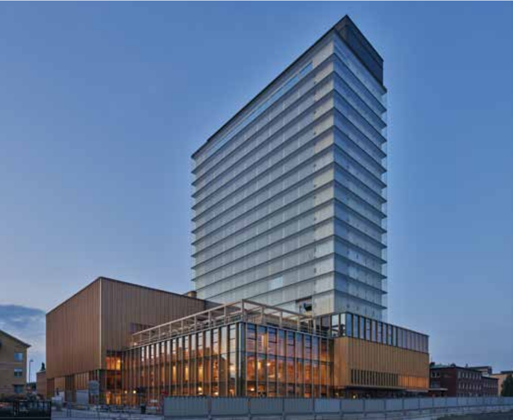
Figure 9. Sara Kulturhus, Skellefteå, Sweden (73 meters, 19 floors), is the world's current tallest steel-timber hybrid building. © White Arkitekter / Åke Eson Lindman
