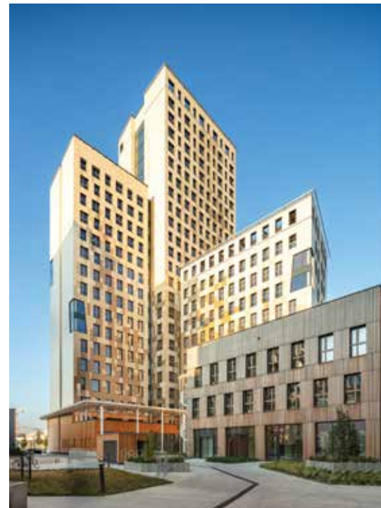
Figure 8. HoHo, Vienna, Austria (84 meters, 24 floors), completed in 2018, is the world's current tallest concrete-timber hybrid building. © DERFRITZ - Fotograf (cc by-sa)
