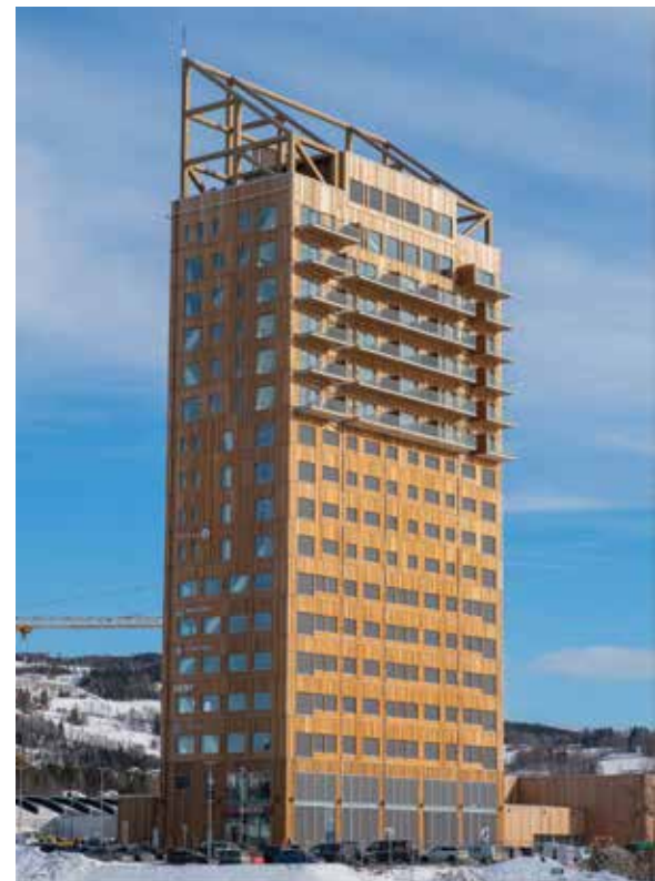
Figure 1. Mjøstårnet, Brumunddal, Norway, is the current world's tallest timber building, at 85.3 meters and 18 floors. © Nina Rundsveen
