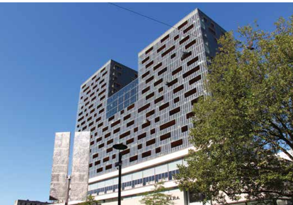
Figure 10. De Karel Doorman, Rotterdam, Netherlands (70.5 meters, 22 floors), is the world's current tallest concrete-steel-timber hybrid structure. The design approach was chosen to facilitate a new residential tower atop an existing 1948 department store. © Fred Romero (cc by-sa)
