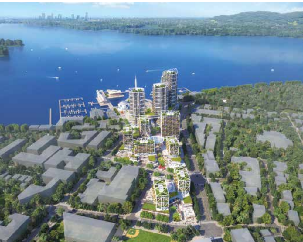
Figure 7. The K2 project seen from the east, with Lake Washington and the towers of downtown Seattle in the background. © Sharkmix
