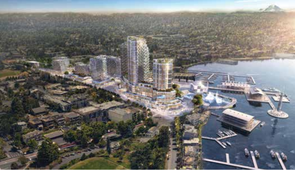
Figure 10. The context, scale, and range of the project, including the aerial gondola system, are shown in this image. © Sharkmix
