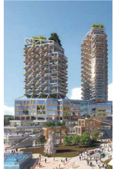
Figure 9. The steel exoskeleton and timber balconies are evident in this view. © Sharkmix
