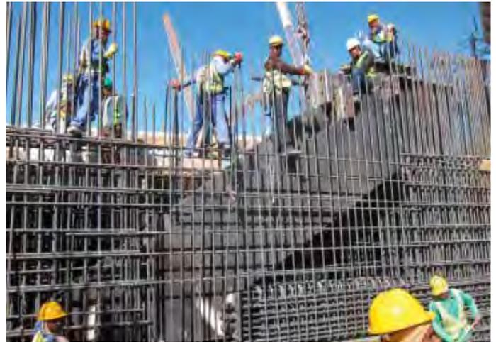
Figure 8. Mega link beam during installation.
