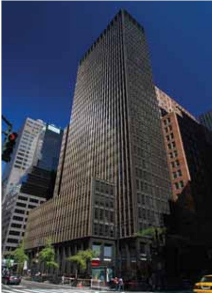
Figure 1. 675 Third Avenue, New York. © Tectonic Photo
