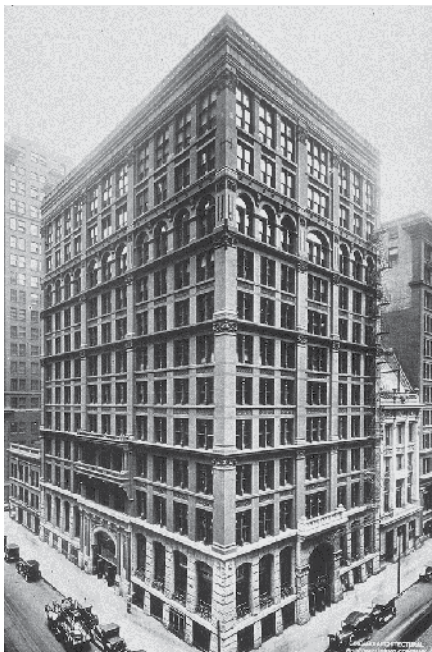
Figure 1. Home Insurance Building, Chicago, 1885.
