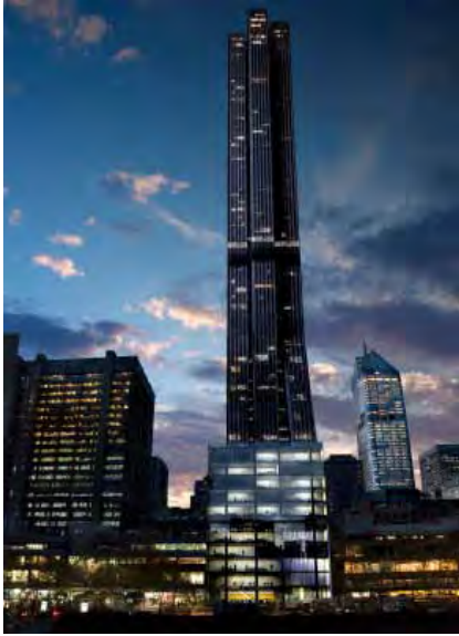
Figure 3. 568 Collins Street, Melbourne, Australia (Source : Stamoulis Property Group / Bruce Henderson Architects)
