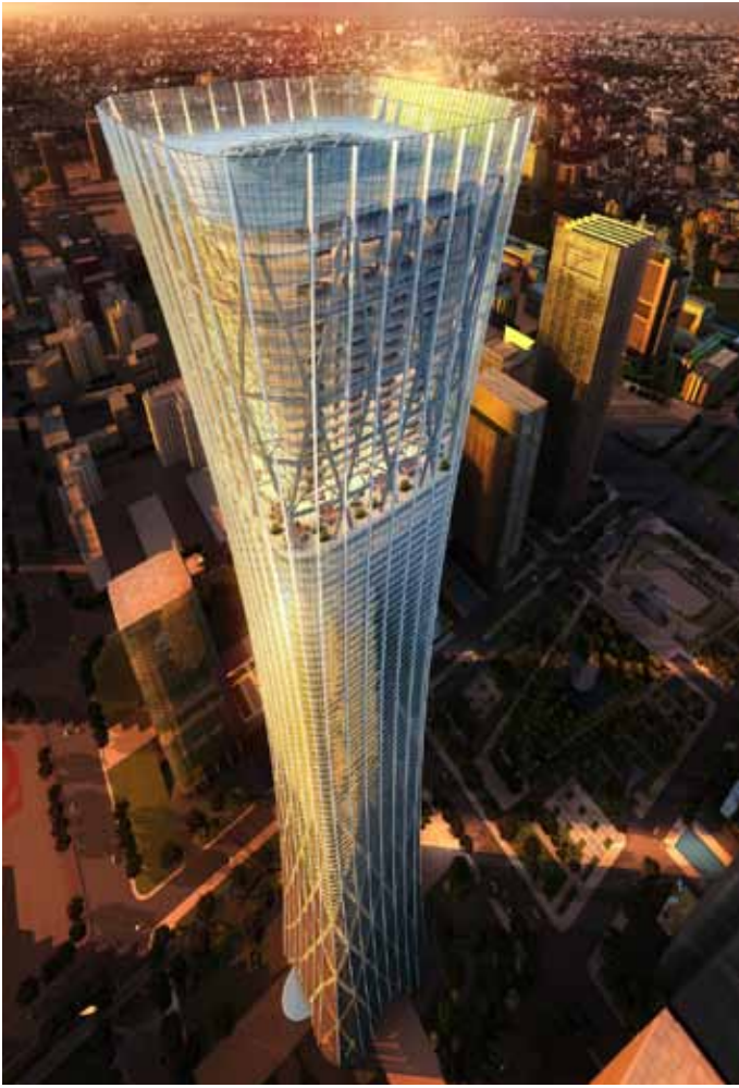
Figure 11. The ancient Chinese vessels inspired Z15 Tower features a distinctive “hour-glass” shape and is reflected in the paths of the southern park to creating a harmony link from the landscape to the tower (Source: TFP Farrells).
