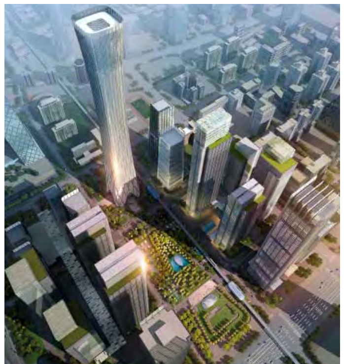
Figure 9. Overview of the mixed-use Beijing Chaoyang District CBD and the Z15 Tower (Source: TFP Farrells).
