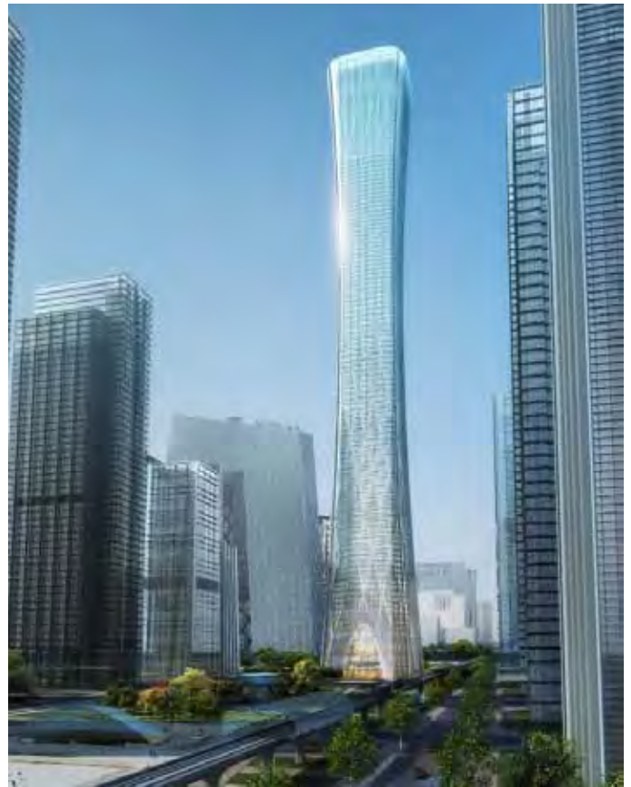
Figure 10. View of Z15 Tower as the focal point of the green spine in the master plan (Source: TFP Farrells).
