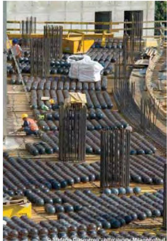
Figure 2. “Bubbledeck” technology. This elements allow a 20% concrete saving if compared to standard solutions. (Source: courtesy of Cobiax)
