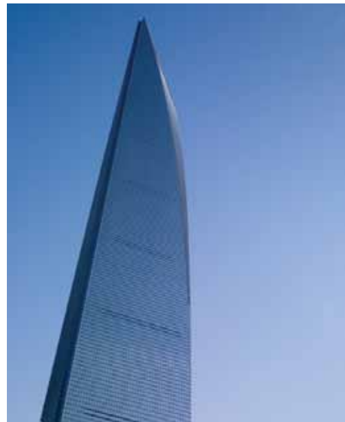
Figure 1. The compact tapering form of SWFC suits internal functions. (Source: KPF. Photography: Tim Griffiths)
