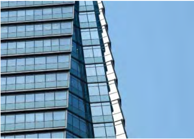
Figure 2. ICC's re-entrant corners improve aerodynamic performance. (Source: KPF. Photography: Tim Griffiths) 图2. ICC凹角处理改善了风气动力学性能（来源：KPF 摄影：Tim Griffiths）
