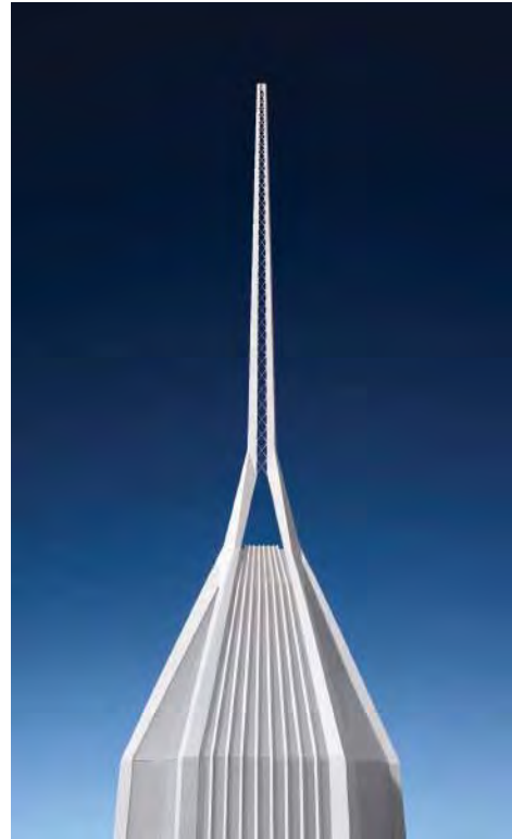
Figure 11. Proposed aerodynamic modifications of the tower spire. (Source: KPF. Photography: Jock Pottle)
